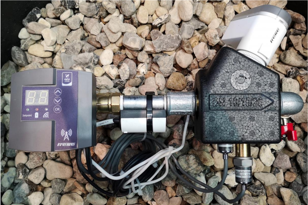
Figure 4: Frese BYPASS installed at Viborg district heating 2
